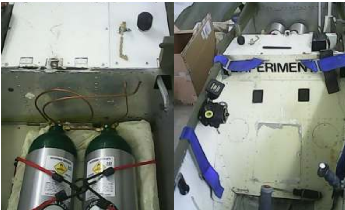
Figure 2 - Installed Oxygen System
